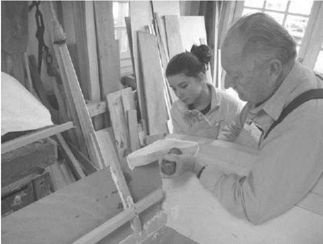
Installing a Quarter knee
